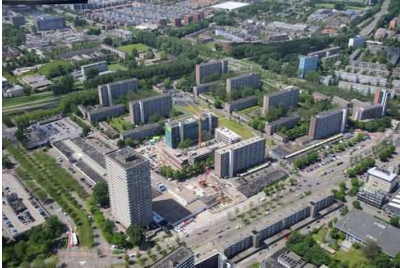
Photo: Renovation project Poptahof, Delft
