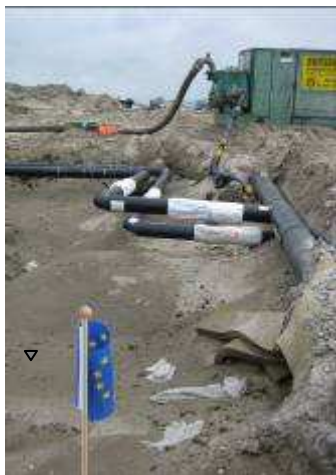
Laying the foundations for grid connection in Harnaspolder, Delft
